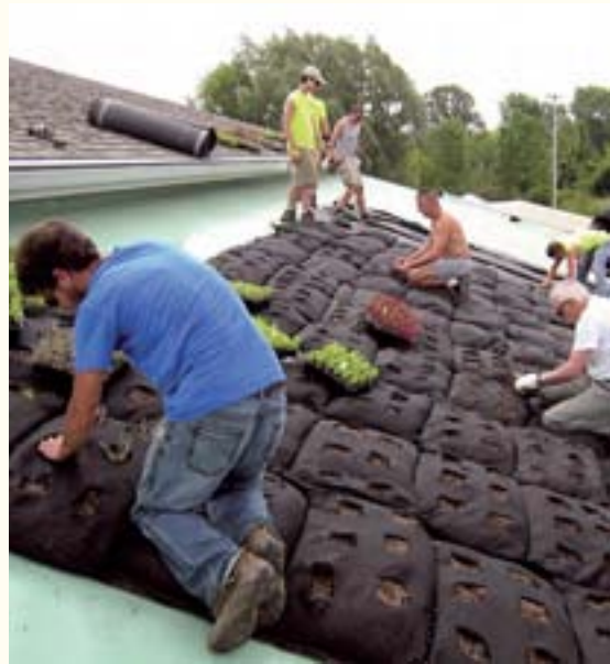
Milwaukee Metropolitan Sewerage District
