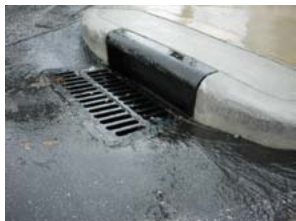
Stormwater Services of Wilmington, NC
